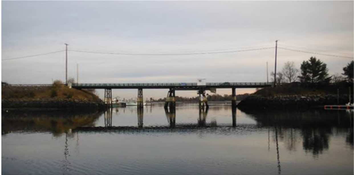
Figure 2. The Wentworth Bridge, looking south. Overhead utility lines shown above the north shoulder.
