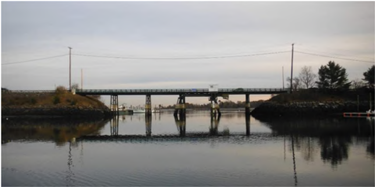
Figure 2. The Wentworth Bridge, looking south. Overhead utility lines shown above the north shoulder.
